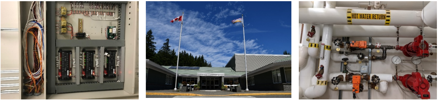
Figure 3 - Huband DDC Systems Upgrade – Building Controls and Control Valves
