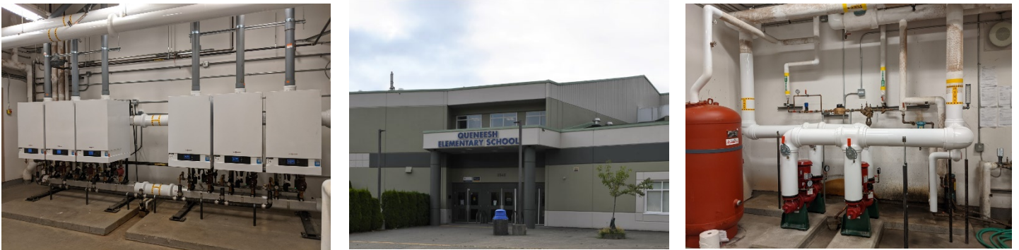
Figure 2 – Queneesh Elementary School Boiler and Pump Replacements
