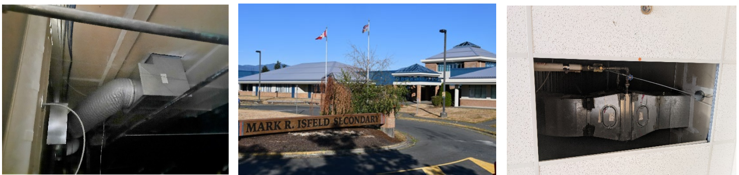
Figure 4 – Mark R. Isfeld Secondary HVAC (mechanical) Phase 2 Upgrades: Ducted Air Return Installed
