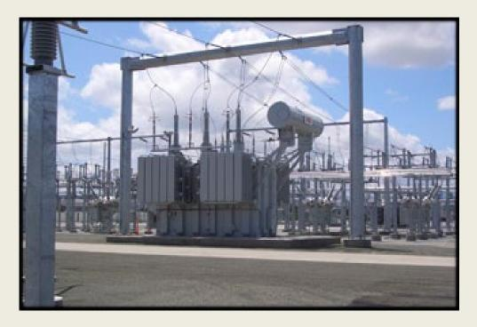
A distribution substation is a system of transformers, meters, and control and protective devices. At a substation, transmission line voltage is reduced to lower voltages for distribution to residential, commercial, and small and medium industrial customers.
