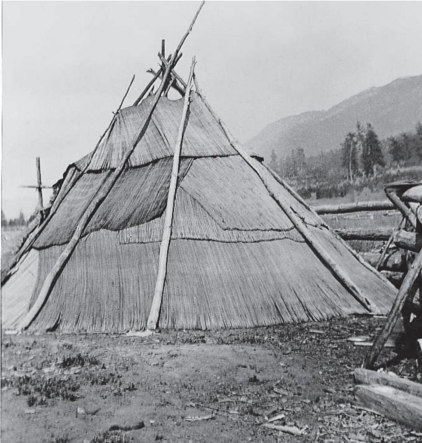
A frame of poles covered with woven mats was a common form of summer housing in the interior, as it allowed for easy movement.
