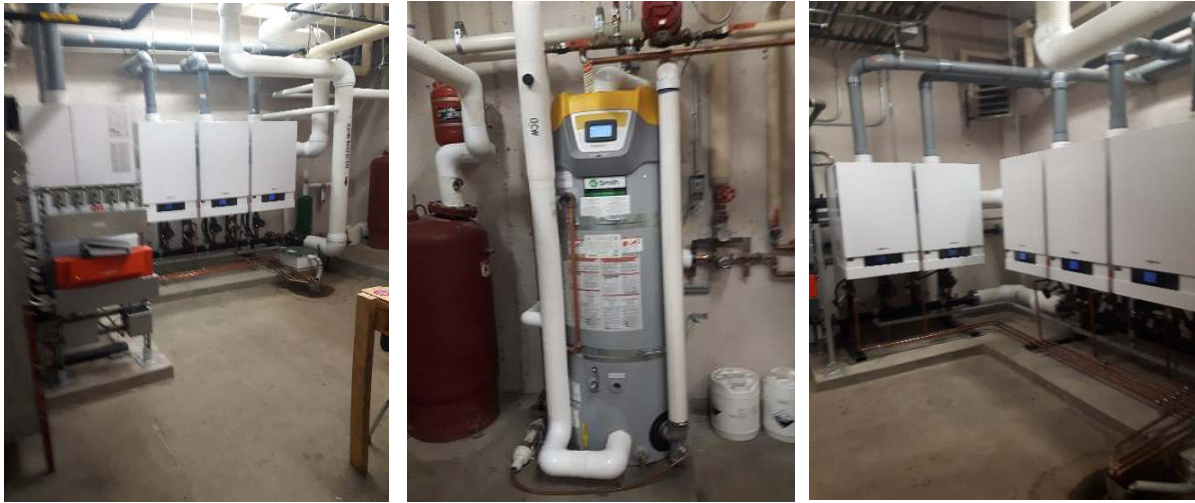
Figure 4 - Valley View School Boilers & Water Heater Replacements (pumps also replaced)
