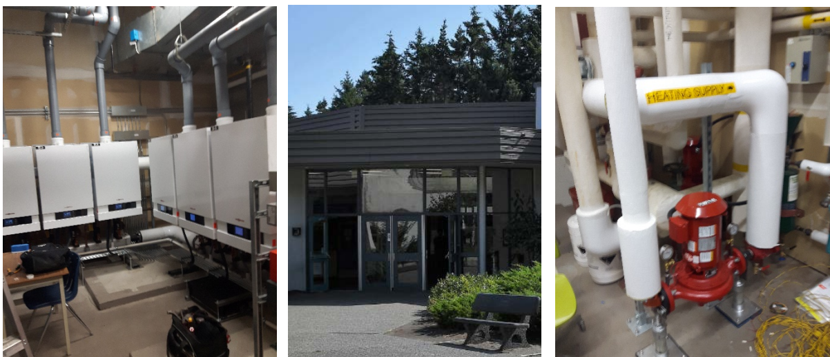
Figure 6 – Highland Secondary Boiler Plant Replacement Project.
