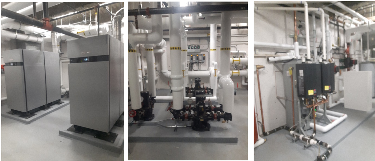
Figure 8 – Mark Isfeld Secondary Boiler Replacement Project.
