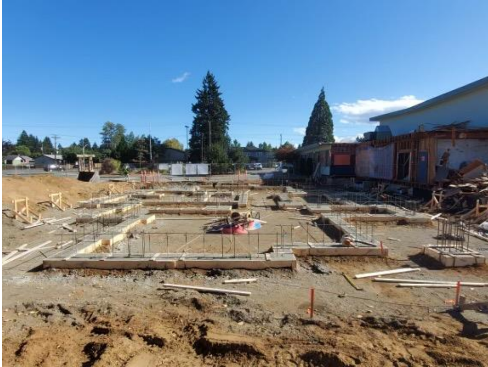
Childcare facility foundation
