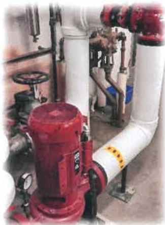
Figure 3- New Pumps installed in Aspen Elementary
