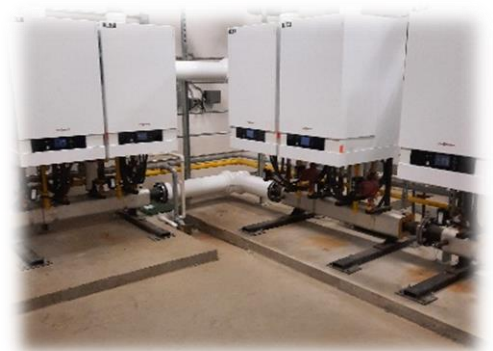
Figure 2 – New boilers installed at Aspen Elementary
