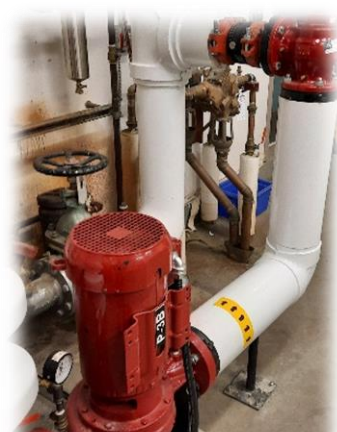
Figure 3- New Pumps installed in Aspen Elementary
