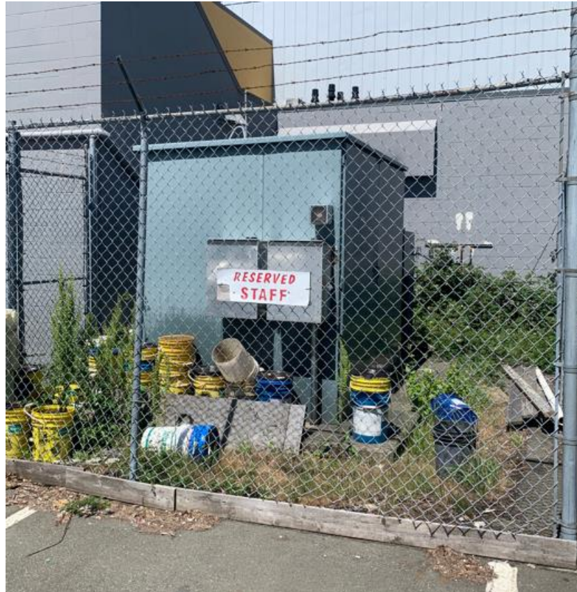
Figure 3: Existing Outdoor Unit Substation
